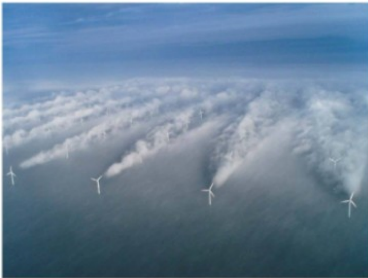
Horns Rev offshore wind farm with turbines in each other's wake
