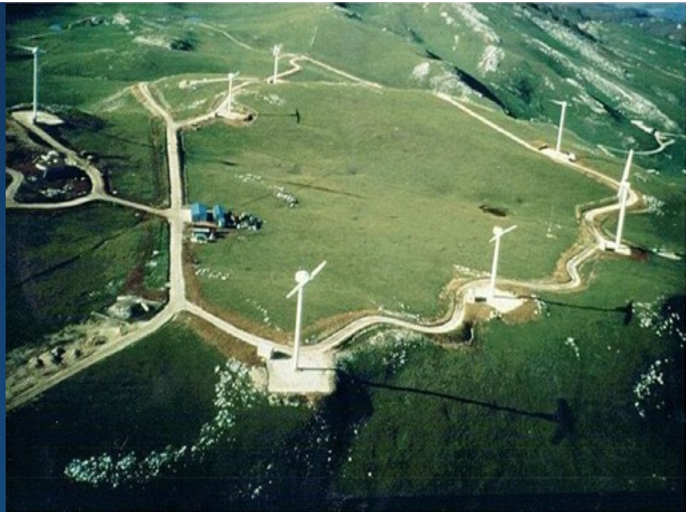
Acqua Spruzza site in Italy
